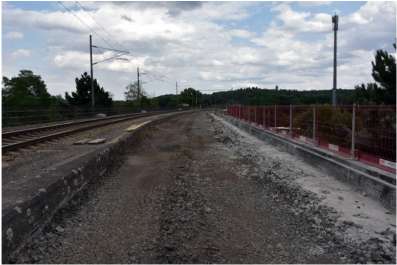
Fig. 19. Locality Prague - Chuchle with damaged plot of Aegilops cylindrica in 2023
